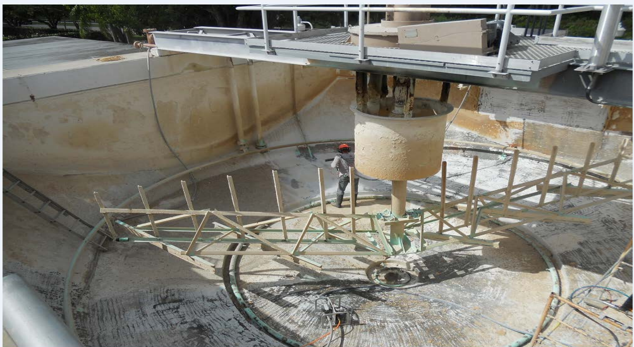
Tank - Before 2SM
