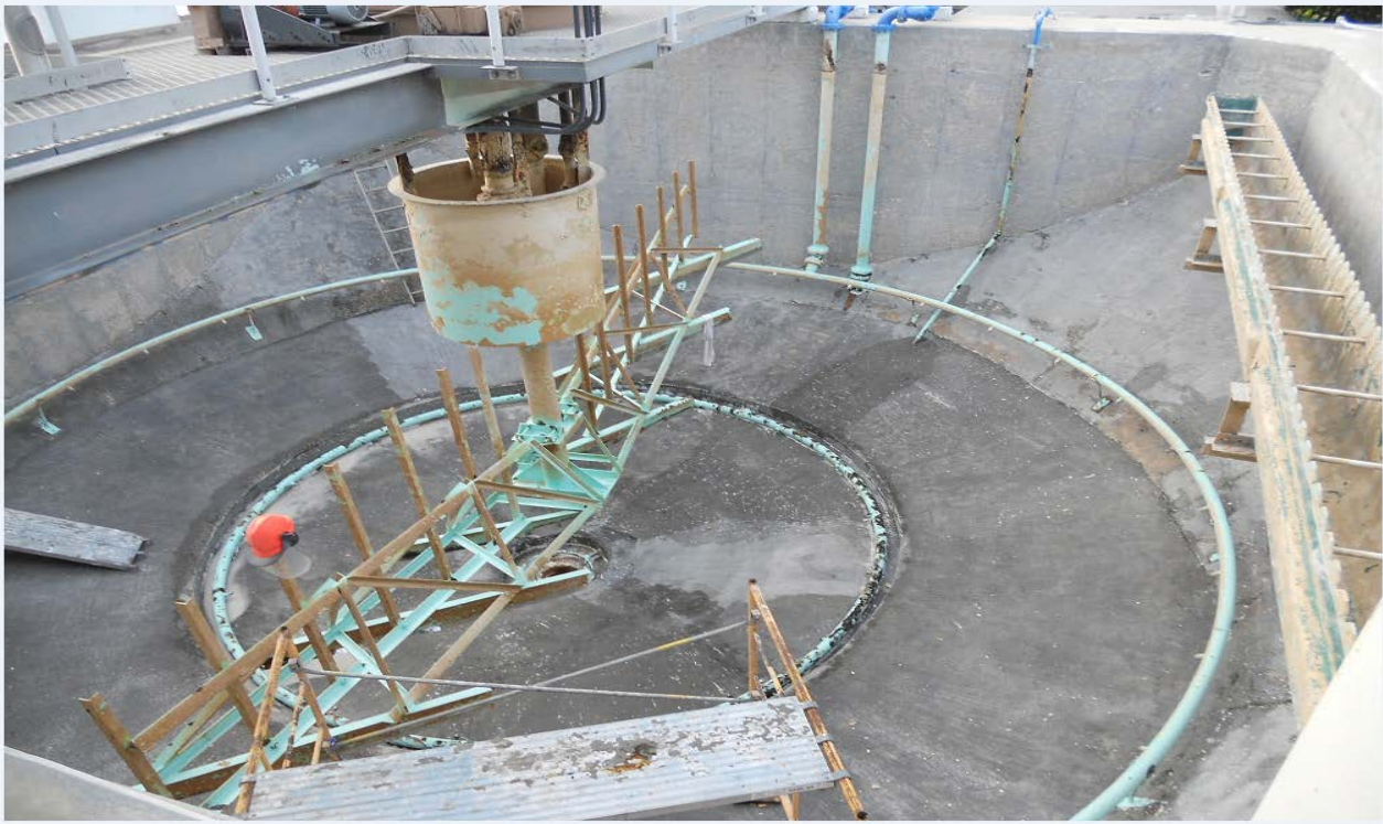
Tank - Before 1SM
